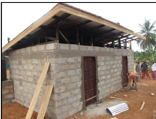
Nearly Completed Latrine
