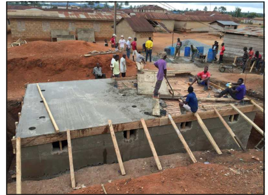
Substructure under Construction
