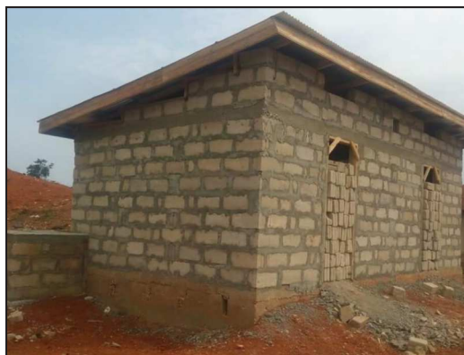
The completed structural portion of the second latrine superstructure. Aesthetic details will be added by the community.
