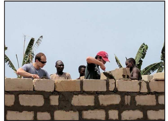
Winter travel team students working with Gomoa Gyaman locals to construct the latrine walls.
