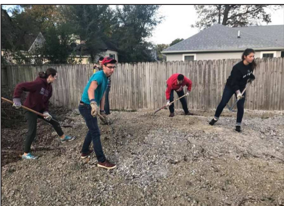
EWB Rose-Hulman volunteers shoveled gravel to create an extended parking lot for a CODA facility in Terre Haute
