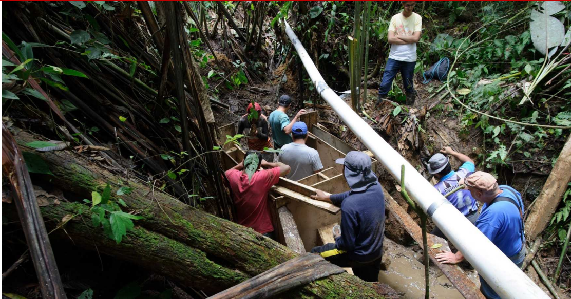
Spring box construction during the March 2020 trip
