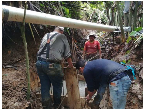
Mentor, Jed Holt, working with local community members on placing the slab on grade for the spring box
